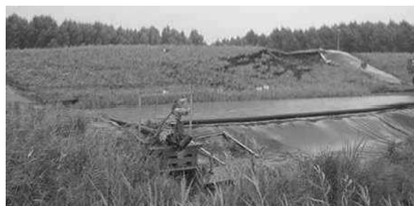
Figure 4. West dike close before failure.
