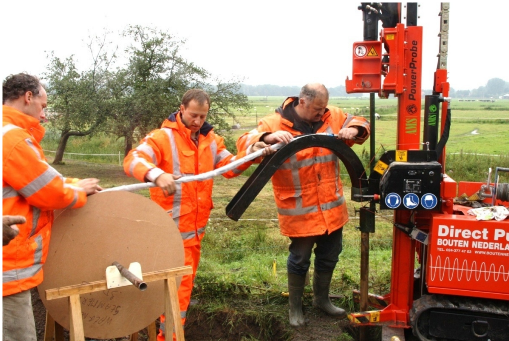
Figure 7: Installation of a GeoBeads string using a light weight direct push-in rig with sonic drilling head.
