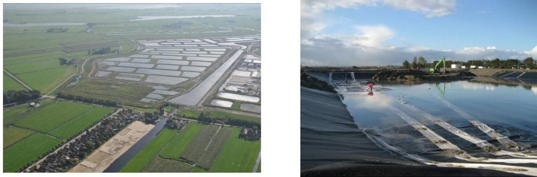
Figure 14. Volgermeer polder (NL) – Aerial view on the left. On the right : the pond lined with a geomembrane and monitored with the TenCate GeoDetect® optical fiber geotextile enabled sensor.
