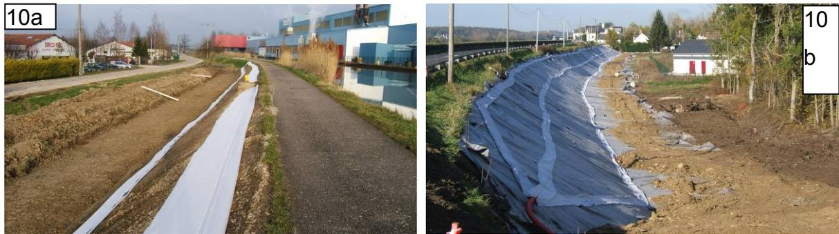
Figure 11. Installation of the fiber optics geotextile enabled sensor along the Marne to the Rhine canal dike (a) and on the flood protection levee along the Loire river / Authion (b).
