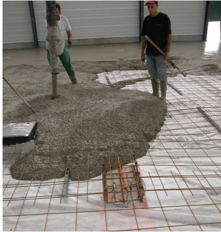
FIGURE 11: Picture of concrete slab pouring when concrete embeds reference sensors.
